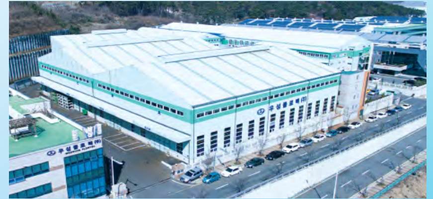
Head office & 1st Factory View
