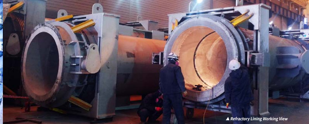
▲ Refractory Lining Working View
