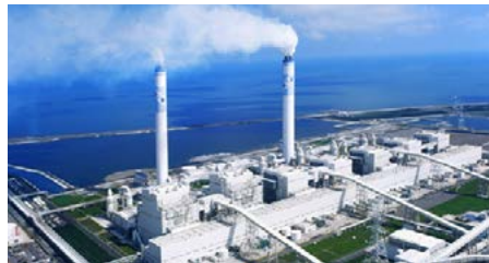
The Mailiao Power Plant is a coal-fired power plant in Mailiao Township, Yunlin County, Taiwan. With a total installed capacity of 4,200 MW, the plant is Taiwan's third-largest coal-fired power plant after Taichung Power Plant and Hsinta Power Plant.
