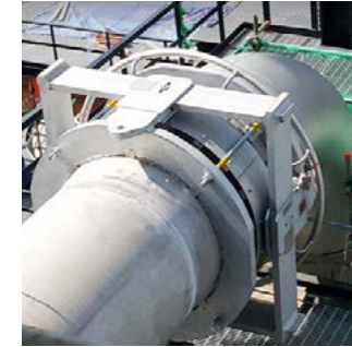
▲ On Site Installation View
