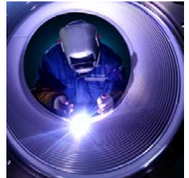
▲ GIS Bellows Welding Work
