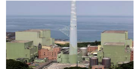
The Lungmen Nuclear Power Plant is a nuclear power plant in New Taipei City, Taiwan. It consists of two ABWRs each of 1,300 MWe net. It is owned by Taiwan Power Company (Taipower).
