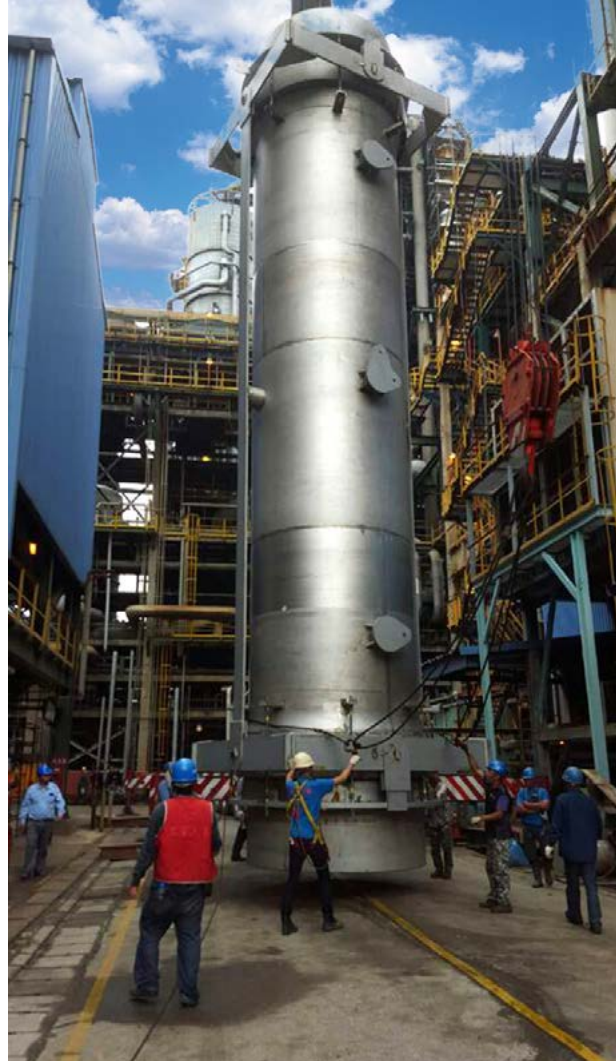
▲ Dual Gimbal Type Expansion Joint
