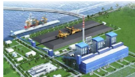
Central Java Power Plant (CJPP) is an ultra critical Coal-fired power plant with 2 x 1,000 MW capacity in Batang Regency, Central Java.
