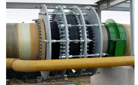
▲ In-Line Pressure Balanced Type Installation View
