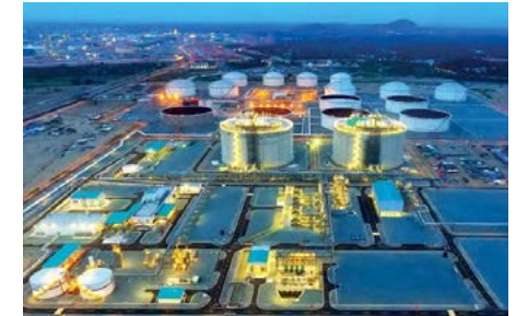
PETRONAS Refinery and Petrochemical Integrated Development (RAPID)
