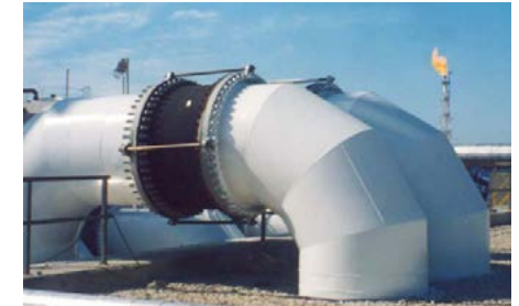
▲ Rubber Expansion Joint Installation View
