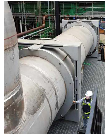
▲ Dual Gimbal Type Expansion Joint installation View
