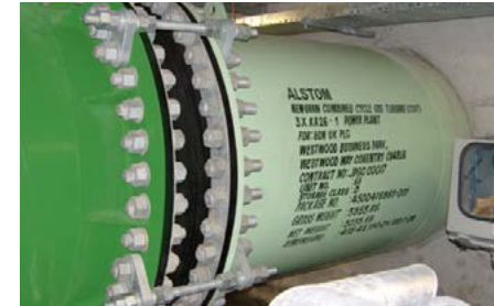
▲ Single Open Arch Type Rubber Expansion Joint
